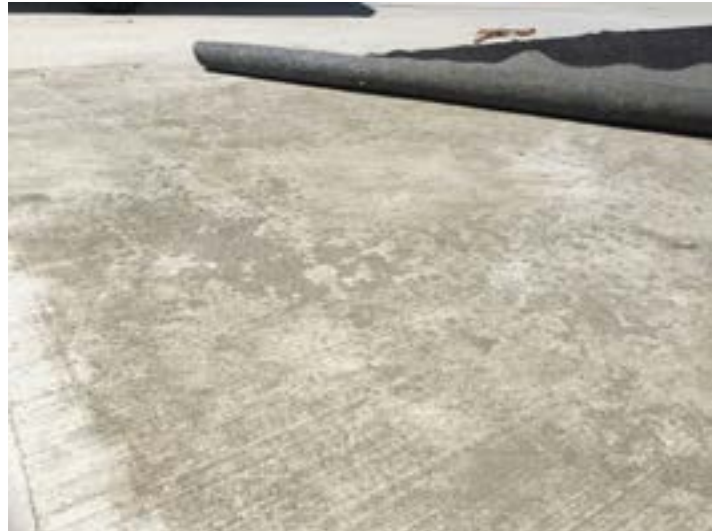
Mats can damage the new docks as seen in this photo.
